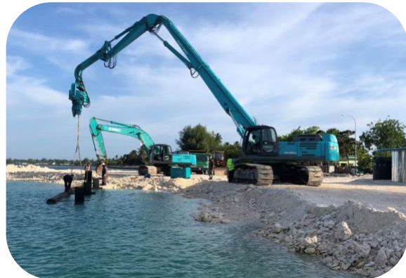
Piling hammers
